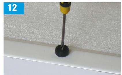
Find the centre point for the post block(s) and pilot drill a 3mm hole. Fix block in position with a No8 x 25mm pan head screws.
