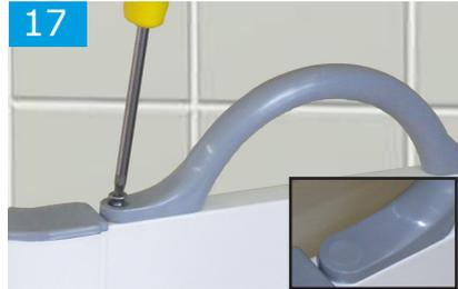
Place door handle(s) against the leading edge of the door(s) on the top rail. Pilot drill the top rail and fix handle to the door with the countersunk self tapping screws. Fit blanking caps, see inset image.
