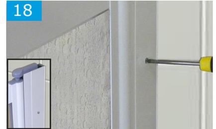
On completion of building the unit, fix the locking screws and caps into both sides of the compensators. Pilot drill two holes to the inside & two holes to the outside of the compensators & secure in position with the supplied pan head screws and grey cover caps, see inset.
