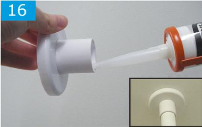
When fitting a floor to ceiling post, first measure from the tray/floor to the ceiling. Now deduct 30mm off your measurement and cut the post to this size. Apply a small amount of silicone sealant to the inside of the ceiling rose collar prior to fitting in place to reduce the amount of play once the post is secured.
