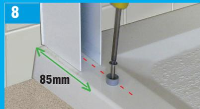
Find the centre point between the compensator. Measure 85mm and pilot drill a 3mm hole. Fix hinge locator to the tray or floor with No8 x 25mm countersunk screw.
