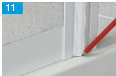
**OPTIONS WITH A VERTICAL SUPPORT POLE:** Insert the panel in the compensator as Step 4, mark around the post(s) to ascertain the location for the post block(s) when the panels are in the correct position.
