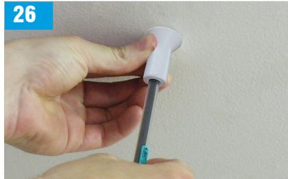
Mark position for the ceiling rose and fix to the ceiling using a suitable fixing (not supplied). Cut drop rod to length.
