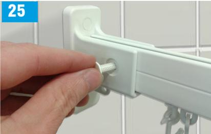
Secure the curtain rail into the wall brackets with the supplied nylon pins. Simply push the pin through the bracket into the holes pilot drilled into the curtain rail.
