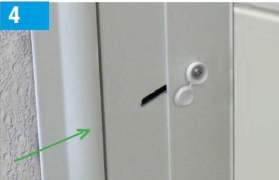
Offer door(s) / fixed panel into their respective compensator ensuring that the slots engage with the adjusting screws. Tighten adjusting screw with the supplied allen key.
