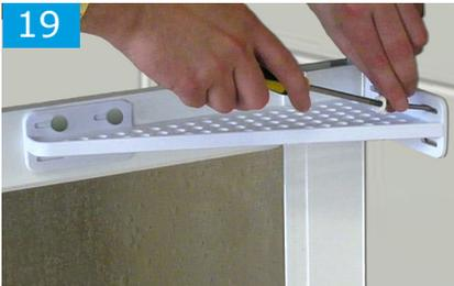
Place panel support bracket against wall and just below the top edge of the top rail (Approx 5mm), on the inside of the enclosure. Mark & pilot drill holes on the rail & wall and fix the bracket in position with the supplied screws and cover caps.
