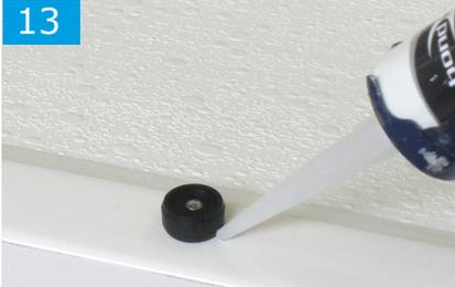
Place a small amount of silicone sealant around the post block(s) and re-fit panel assemblies in position. Fully tighten compensator adjusting screws to secure in position, as shown in Step 9.
