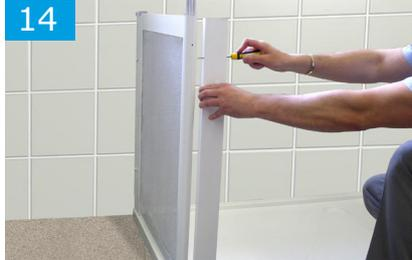
If fitting a post compensator, inline or off a return panel, place the compensator against the post and mark through the fixing slots. Find the centre of your mark and drill a 3.8mm dia hole. Fix in place with No8 x 25mm pan head self tapping screws. Offer door into post compensator as described in steps 4 to 8.
