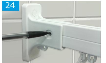
Place curtain rail into wall brackets. Mark holes onto curtain rail through wall bracket on both sides and pilot drill rail with a 4.5mm diameter drill.
