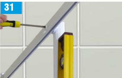
Ensuring the post is straight, pilot drill through both the curtain rail and post using a 3.0mm drill. Screw both together with a No8 x 38mm pan head screw and cap.
