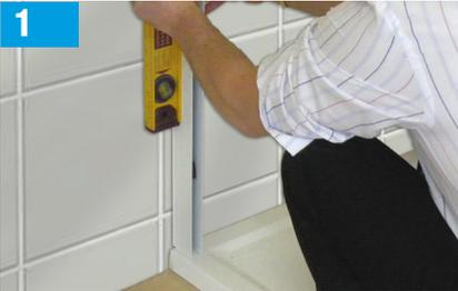
Place compensators against the wall ensuring that they rest on the flat area of the tray or floor at the position shown. Mark off fixing holes on the wall when level.
