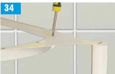
Screw the boomerang bracket to the curtain rail using the No6 x 3/4" countersunk screws. **USE THE SCREWS PROVIDED.**
